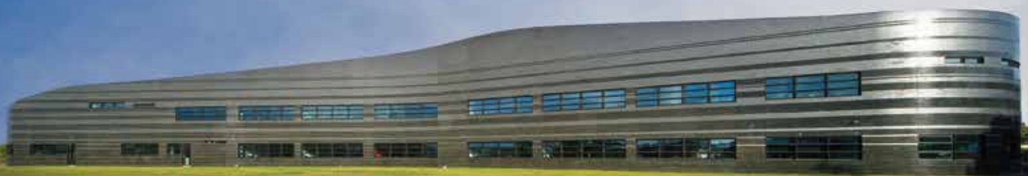
The building is clad in gloss-black and silver-banded brickwork, like a medieval walled city.
